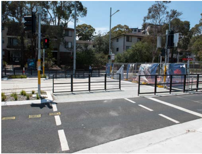
Figure 61. Signalised crossing across a single travel lane with balustrade dog-leg (PLR, Benaud Oval)
