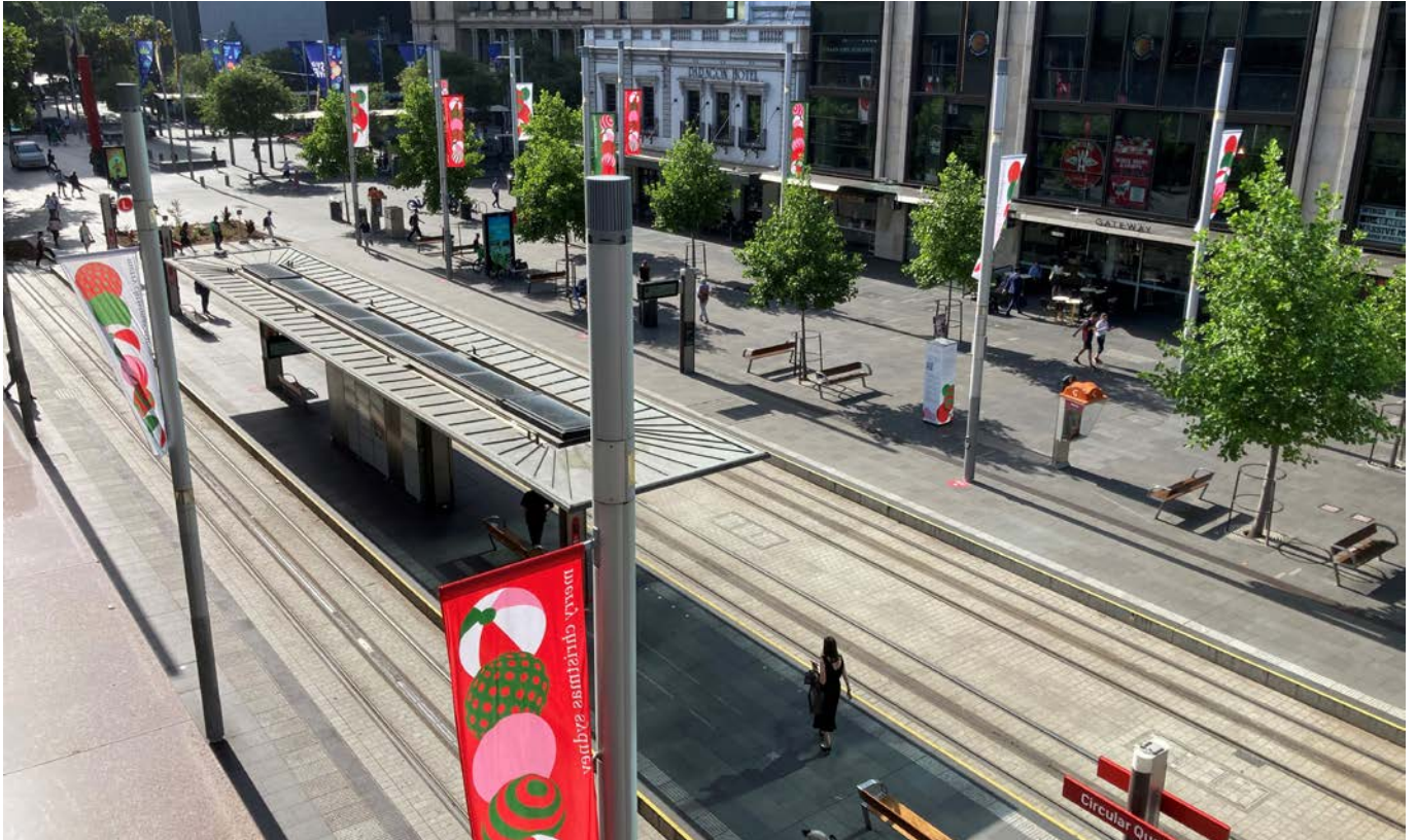
Figure 50. Circular Quay is a multi platform terminus stop with direct level access to the surrounding precinct (CSELR)
