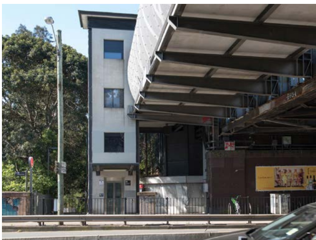
Figure 87. Lift access to elevated light rail stop (IWLR, Marion)
