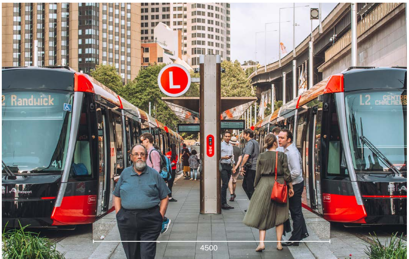
Figure 97. Minimum platform width (CSELR, Circular Quay)
