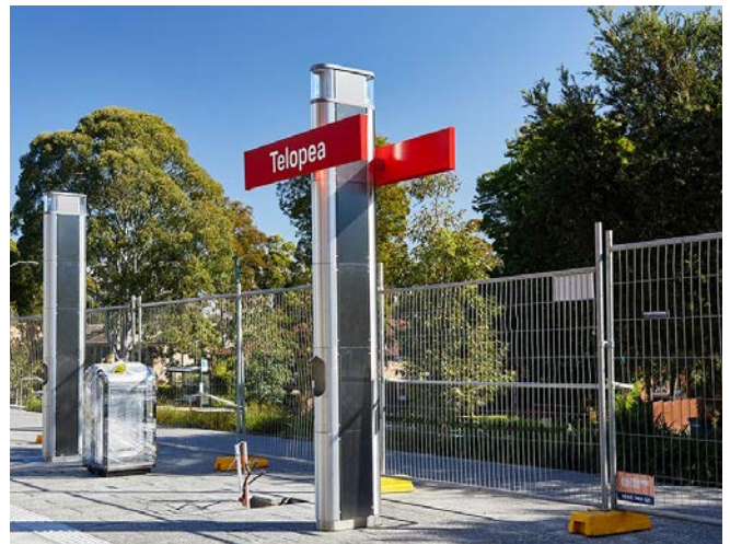
Figure 202. Stop name signs attached to multi-use totem (PLR, Telopea)
