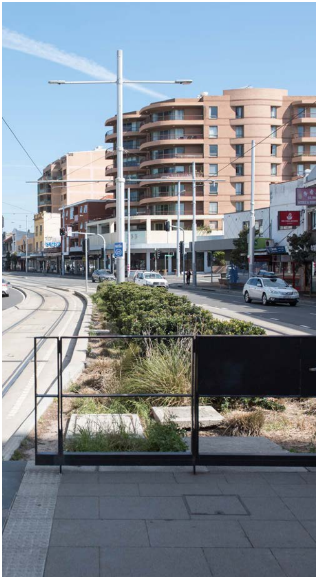
Figure 223. Balustraded end of platform rather than long walkway to next junction
