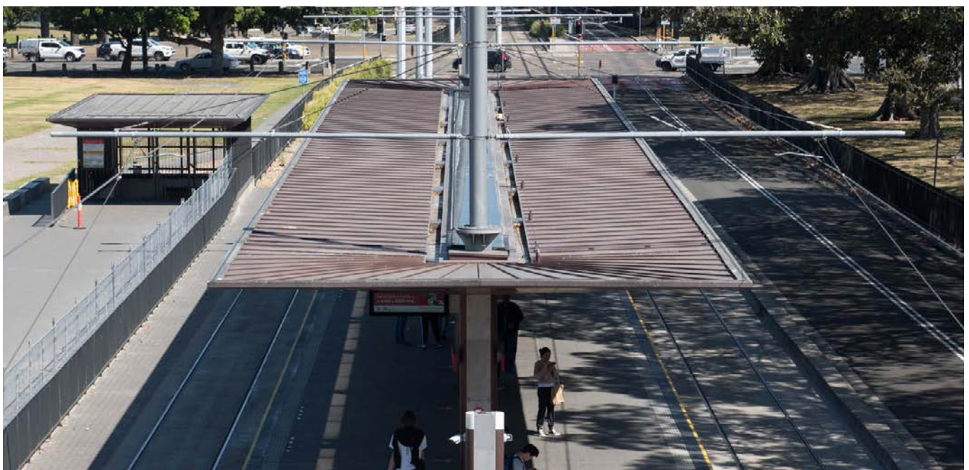
Figure 139. 8000mm canopy module at Moore Park stop to cater for large crowds during events (CSELR)
