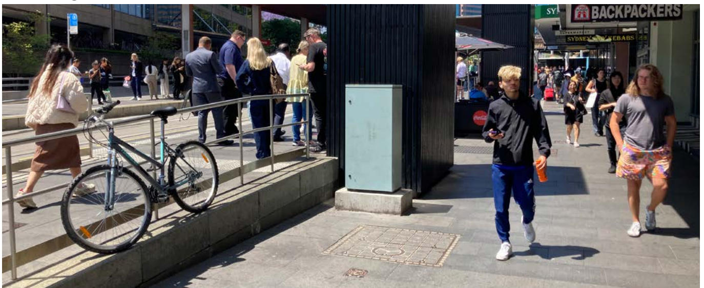
Figure 218. Raised stop level required extra steps, ramps and balustrades to existing footpath
