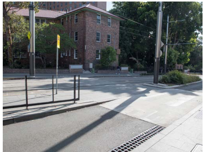
Figure 64. Non-signalised, pedestrian crossing over single travel lane (CSELR, Surry Hills)
