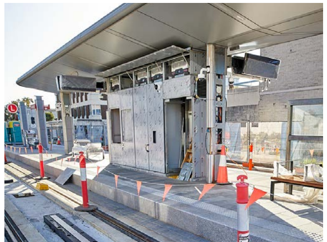
Figure 157. 5 module services cabinet during installation (PLR)
