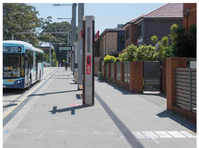
Figure 193. Side platform with same footpath and platform paving (CSELR)
