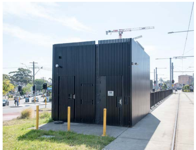
Figure 93. Drivers' facilities as stand alone building (CSELR, Juniors Kingsford)
