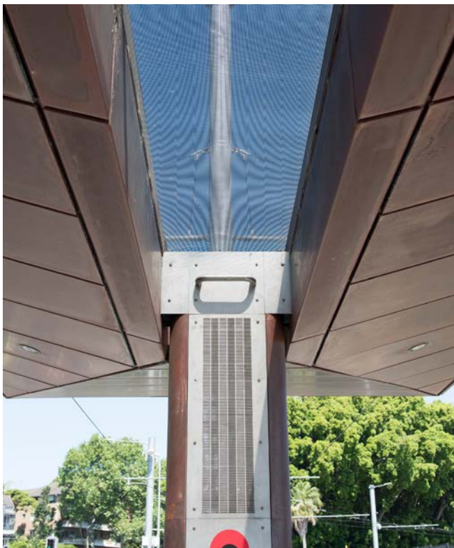
Figure 169. Maintenance access to canopy roof through skylight (CSELR, Wansey Road)
