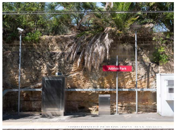
Figure 159. A non integrated solution leads to a cluttered platform (IWL, Jubilee Park)
