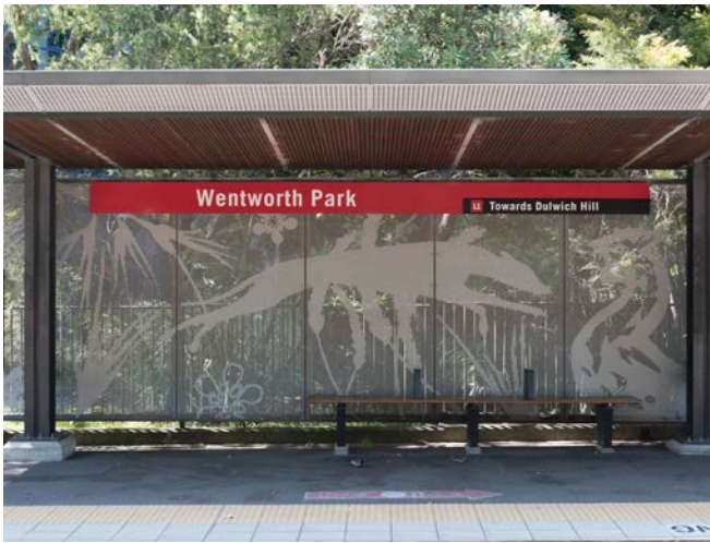
Figure 199. Stop name and direction of travel sign placed in canopy structure (IWLRL, Wentworth Park)
