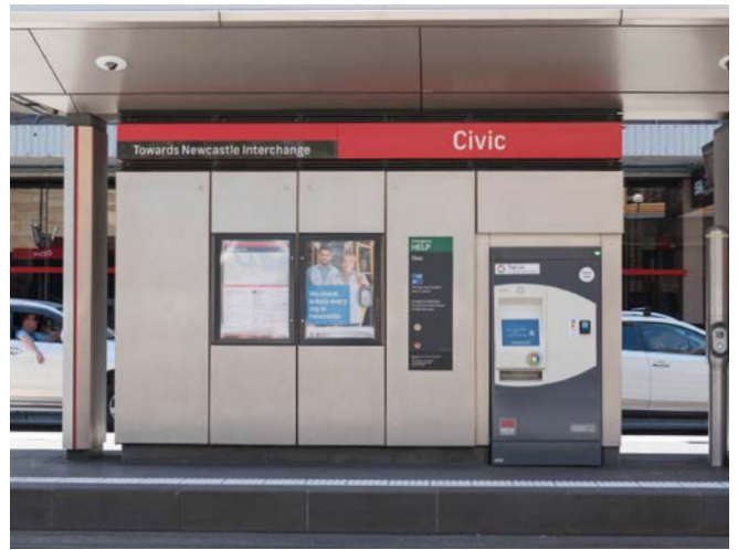
Figure 155. 5 module services cabinet (NLR, Civic)
