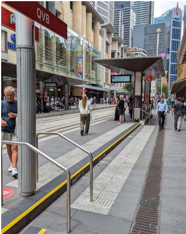
Figure 215. Level transition was not possible due to underground elements
