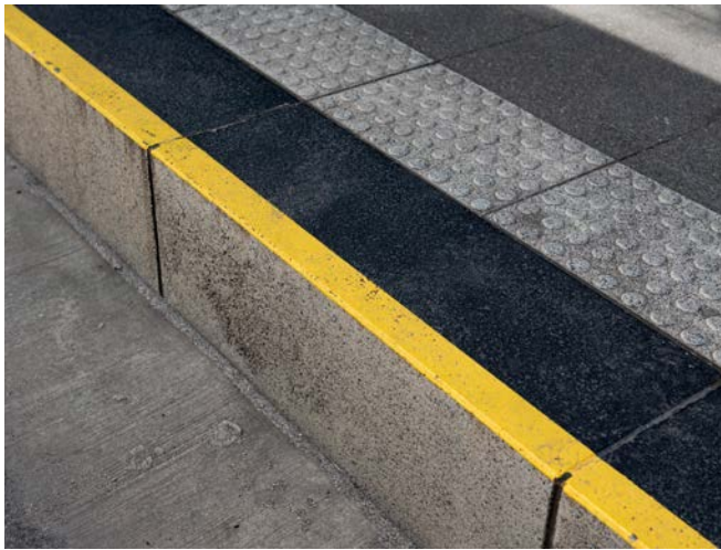
Figure 188. Yellow line retrofitted to coping stone (CSELR)
