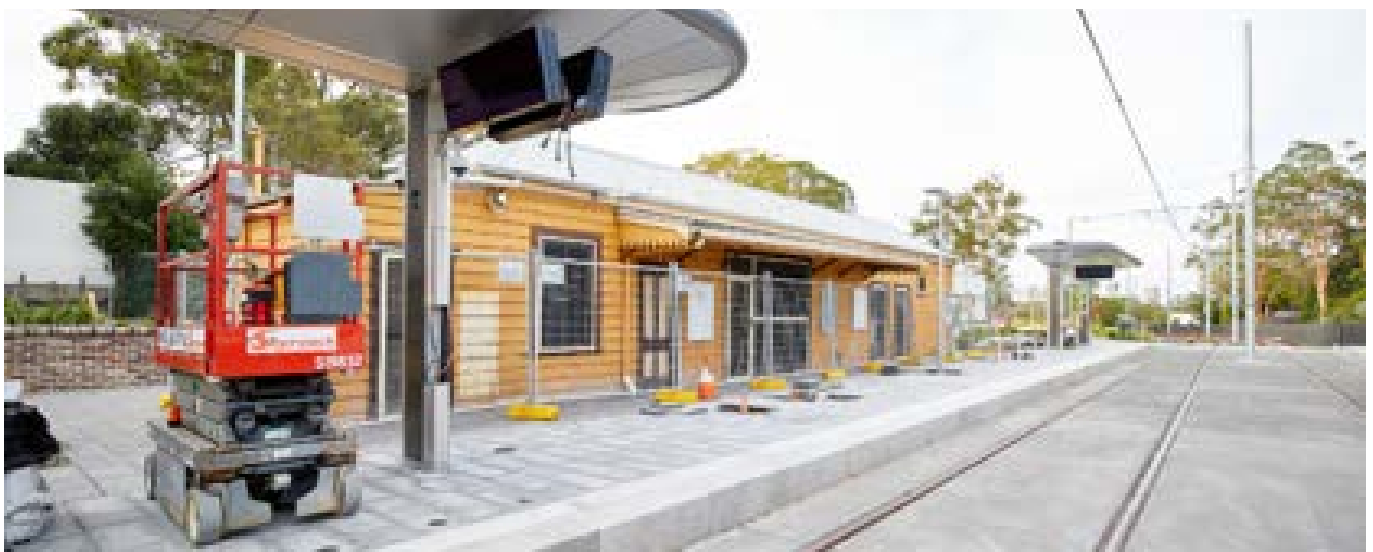
Figure 231. Heritage station framed by the two stop canopies
