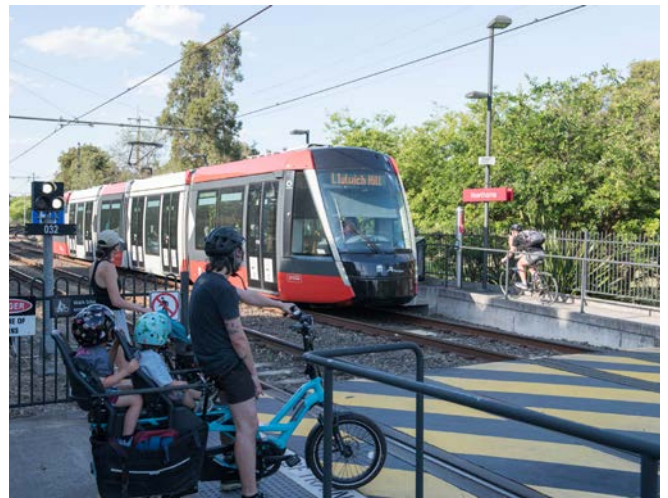
Figure 68. Crossing over ballasted track between side platforms (IWL, Hawthorne)
