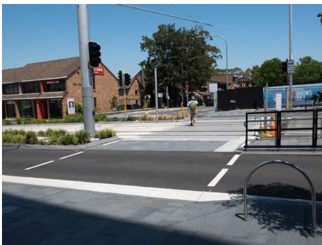
Figure 65. Signalised crossing across the full road reserve (PLR, Fennell Street)
