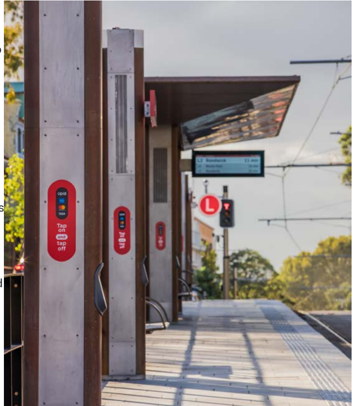
Figure 150. Totems with integrated equipment (CSELR, Surry Hills)
