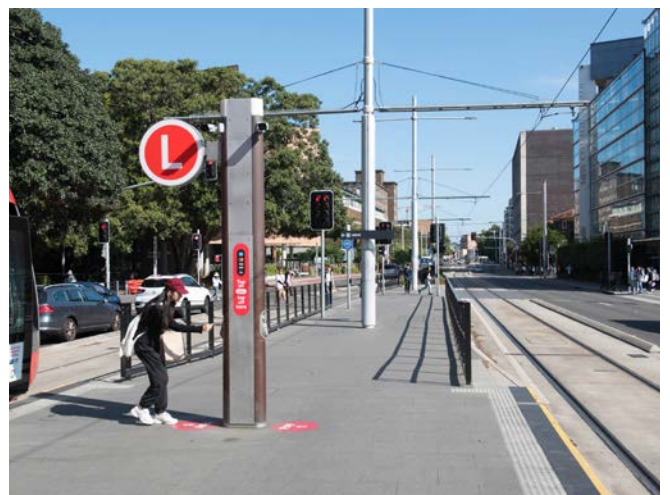
Figure 88. Long ramp from platform to road crossing (CSELR, UNSW High Street)
