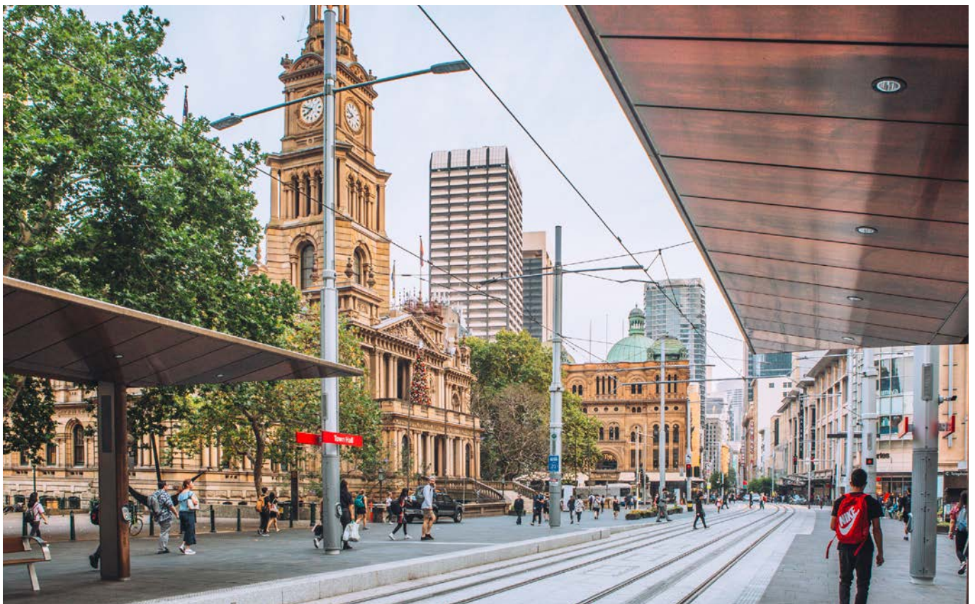
Figure 125. Example of a CSELR stop canopies in relation to heritage context. (CSELR, Town Hall)
