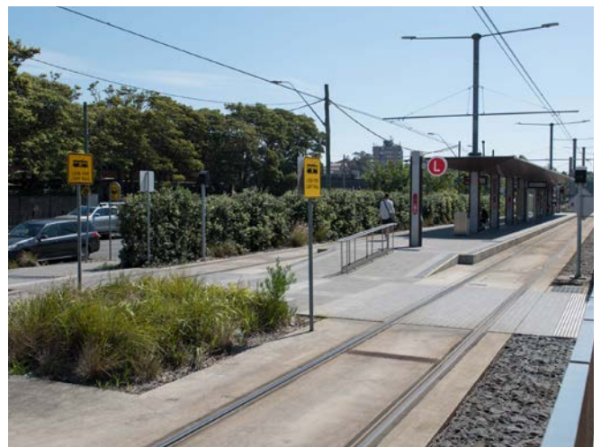
Figure 70. Double track crossing (CSELR, Royal Randwick)
