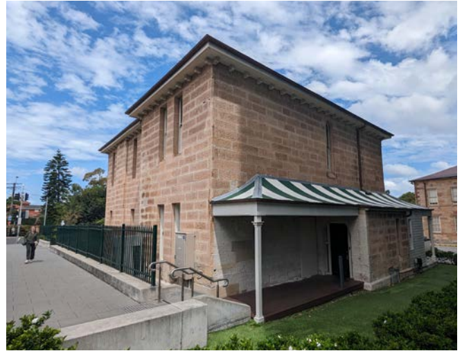
Figure 92. Drivers' facilities integrated into heritage building (CSELR, Randwick)
