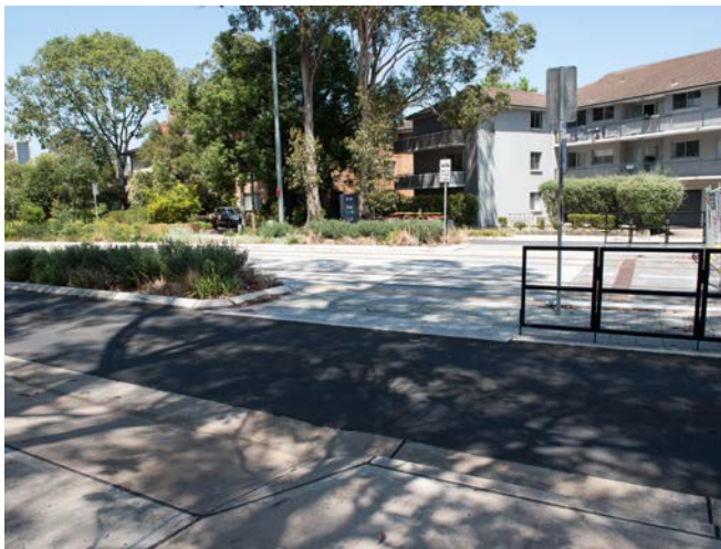
Figure 63. Non-signalised crossing across single travel lane (PLR, Benaud Oval)
