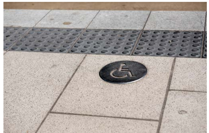
Figure 117. Accessible door marking on Newcastle Light Rail
