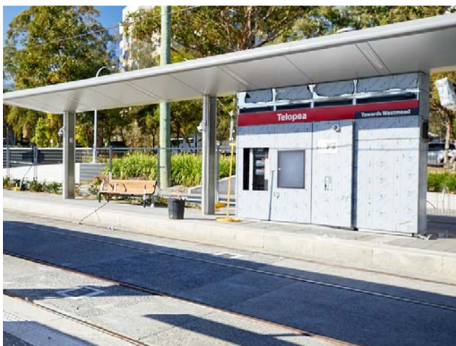
Figure 158. 4 module services cabinet during installation (PLR, Telopea)
