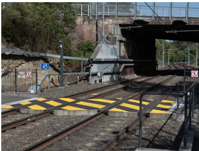
Figure 69. Crossing over ballasted track between side platforms (IWL, Waratah Mills)
