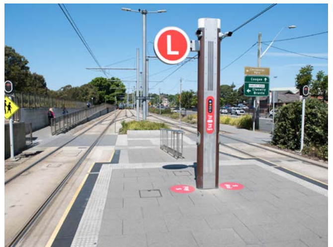
Figure 86. Ramp from pedestrian median with central handrail (CSELR, Royal Randwick)
