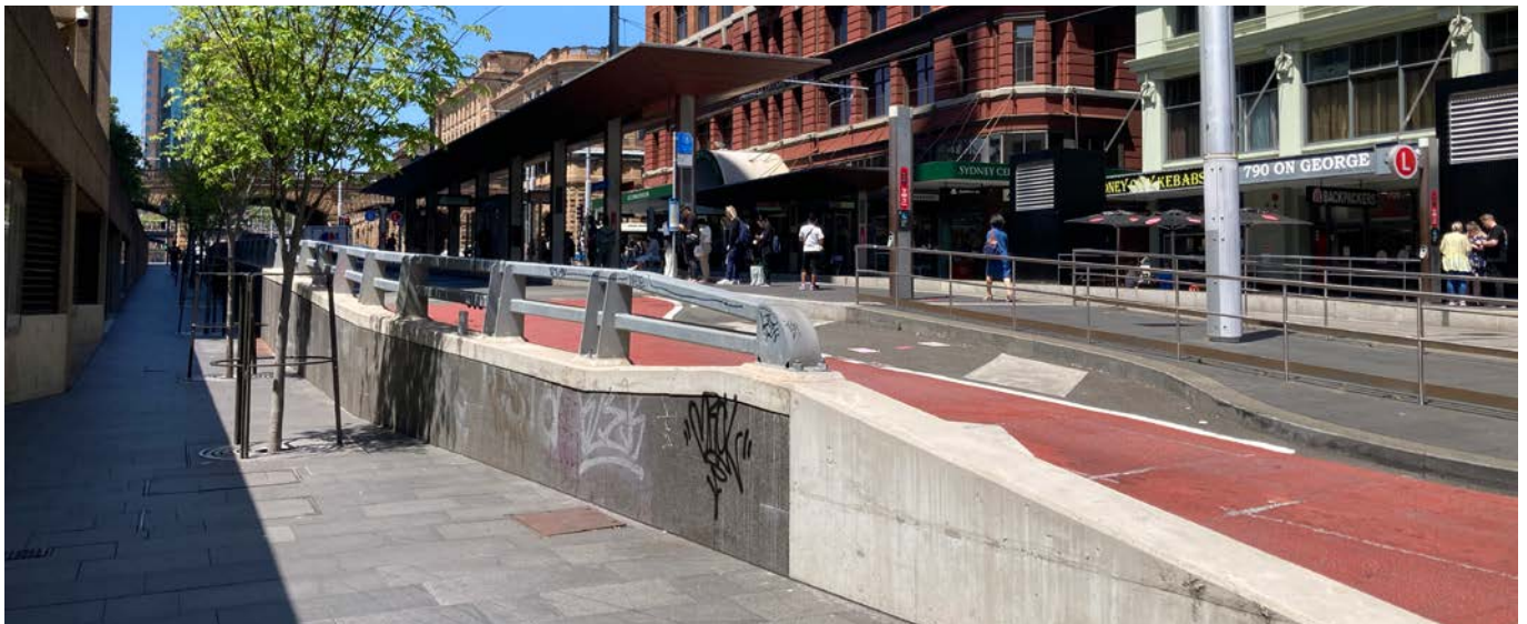
Figure 217. While not a positive footpath outcome, earlier design attention to the barrier wall could have integrated public art or seating
