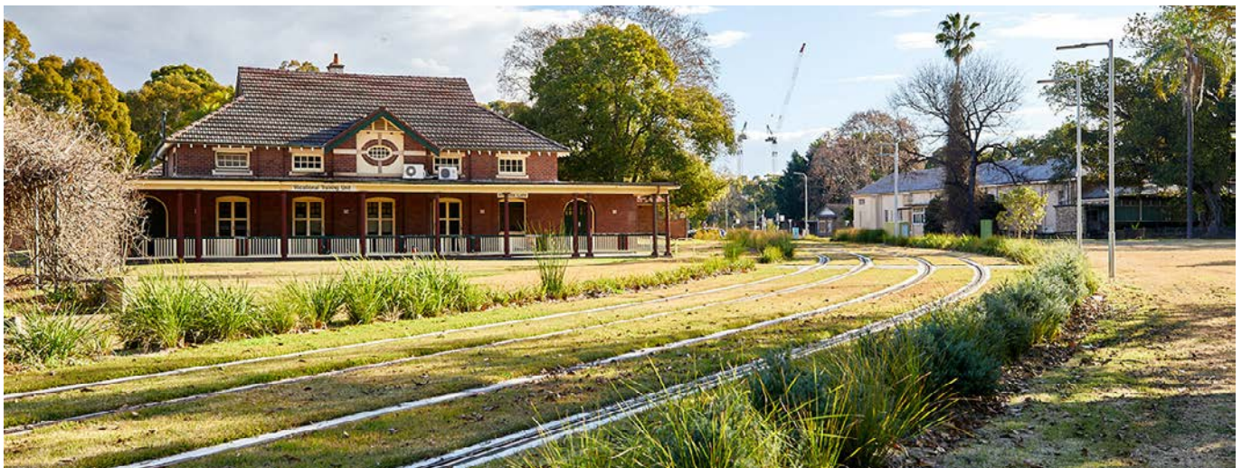
Figure 23. The green tracks assist contextual integration, water permeability and treatment of stormwater runoff (PLR, Cumberland Hospital Precinct)
