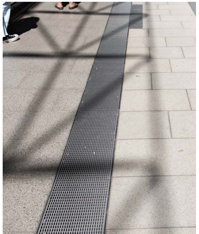
Figure 170. Platform drainage channel recessed into surface (NLR)
