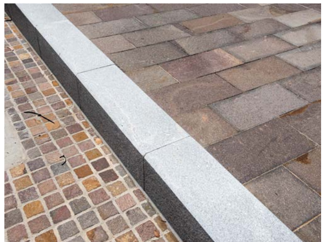
Figure 191. Special paving of track zone in heritage precinct (PLR)
