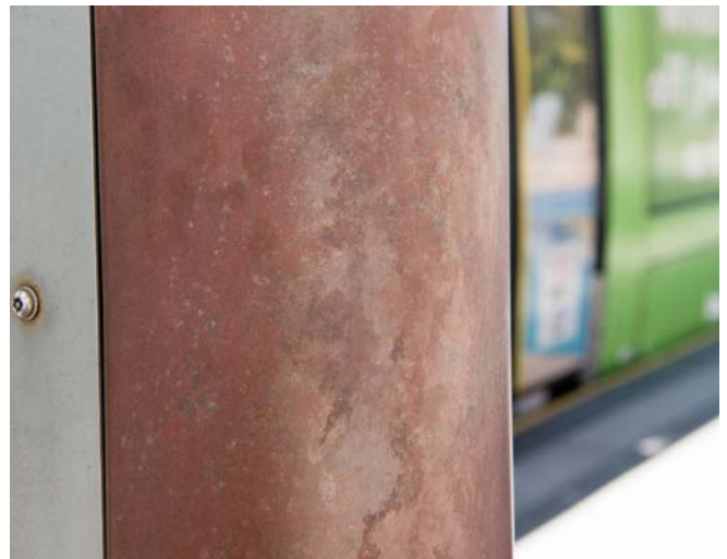
Figure 25. Copper finishes were used on CSEL R for its durability and low maintenance
