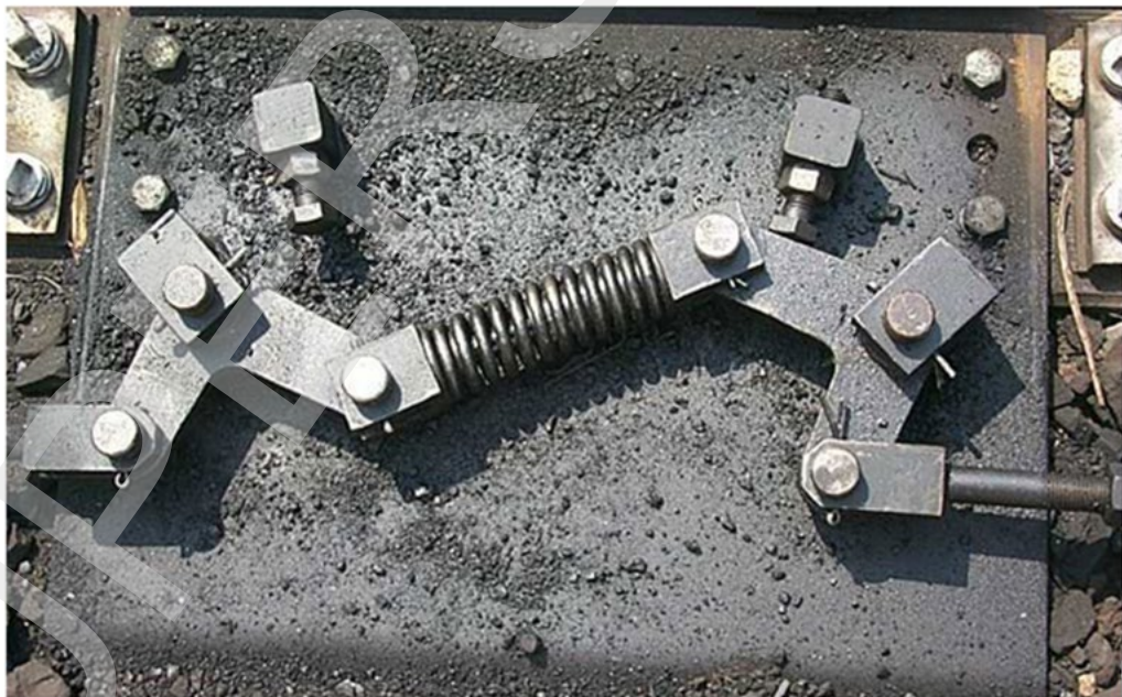
Figure 26 – Spring assist unit
