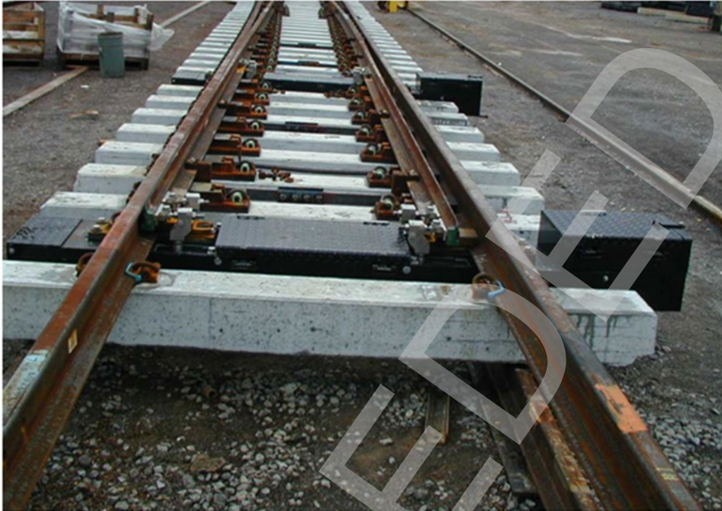
Figure 27 – Separate mechanisms for front and back drives
