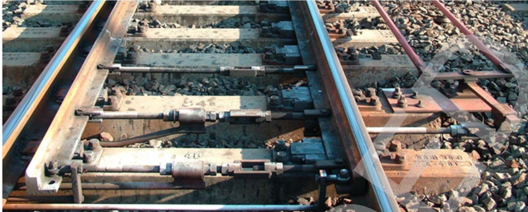
Figure 25 – Mechanical T crank back drive
