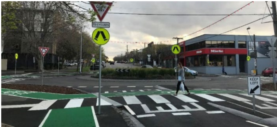
Figure 10 – Cyclists and pedestrian protected roundabout in South Melbourne (Source: Austroads, AP-R611-20)
