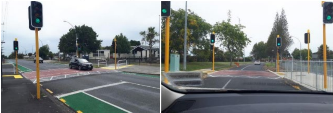
Figure 11 – Raised midblock signalised crossing on Pukete Road in Hamilton, New Zealand (Source: Austroads AP-R642-20)
