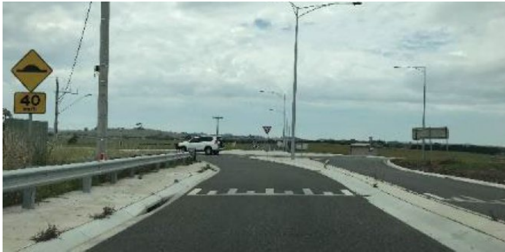
Figure 9 – Raised compact roundabout at Lance Creek, Victoria (Source: Austroads, AP-R642-20)
