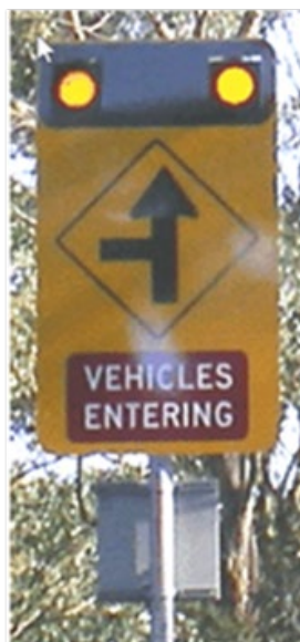
Figure 7 – Example 2 of alternative forms of RISZ that should not be used in NSW (Source Bradshaw et al., 2013, Vehicle Activated Signs: An emerging treatment at high-risk rural intersections )
