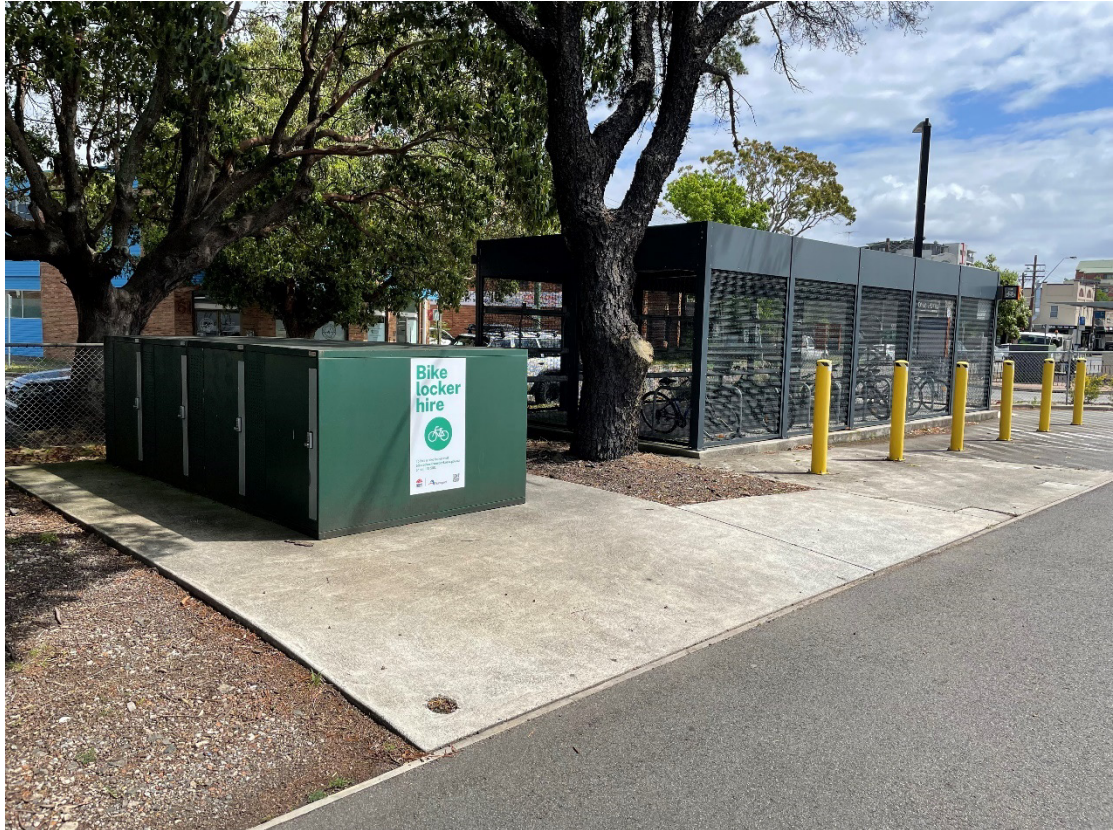
Figure 6 – Co-located bike lockers and a bike shed
