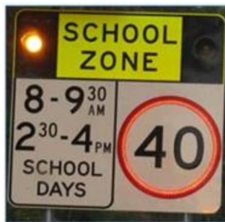
Figure 48 – Flashing school zone sign – with annulus
