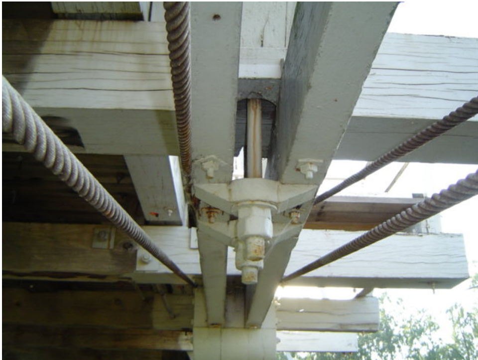
Tie rods in good condition.
