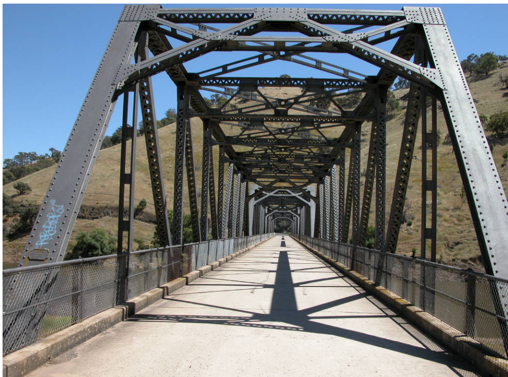
Element in new or near new condition.
