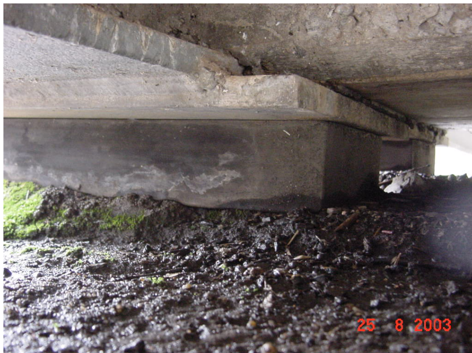
Elastomeric bearing in good condition. General cleaning required.
