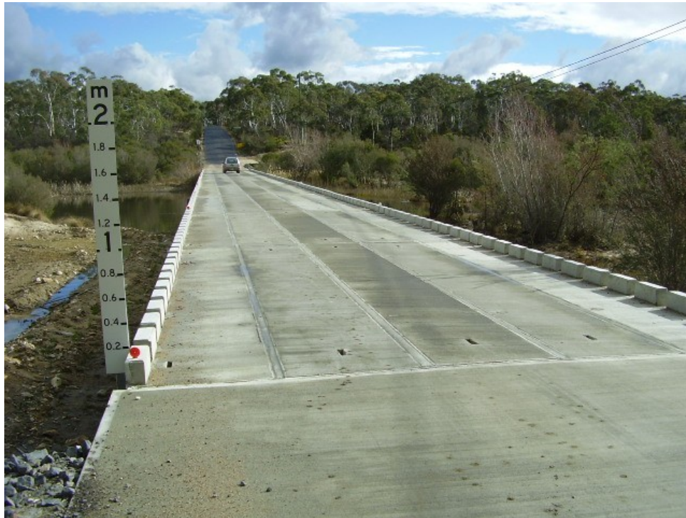
Approach carriageway in good condition.
