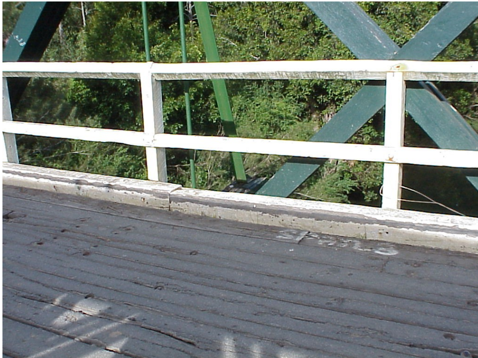
Timber railing in good condition.
