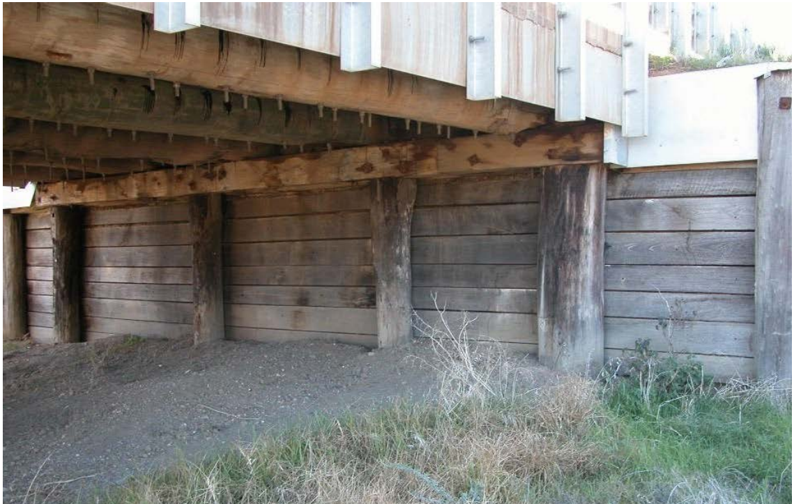
Abutment sheeting in good condition.
