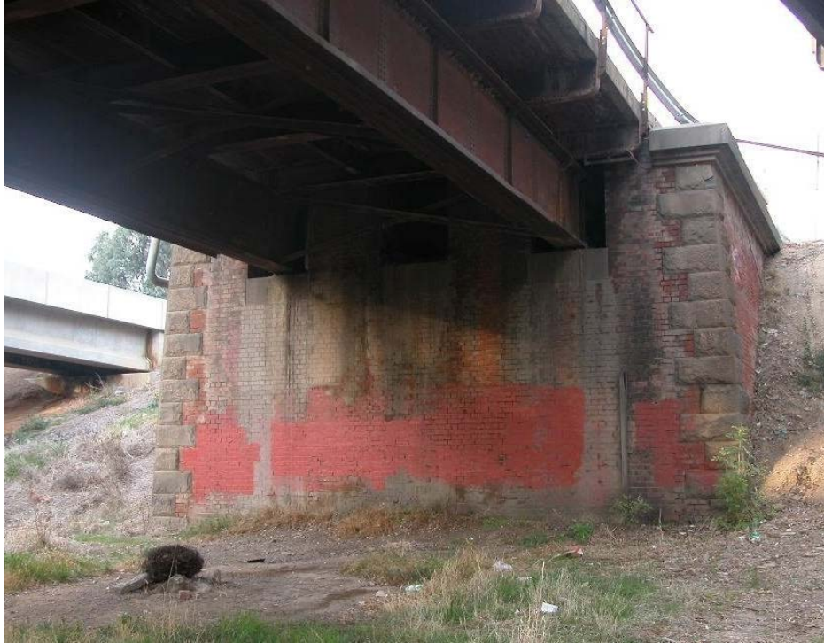
Masonry abutment on good condition.
