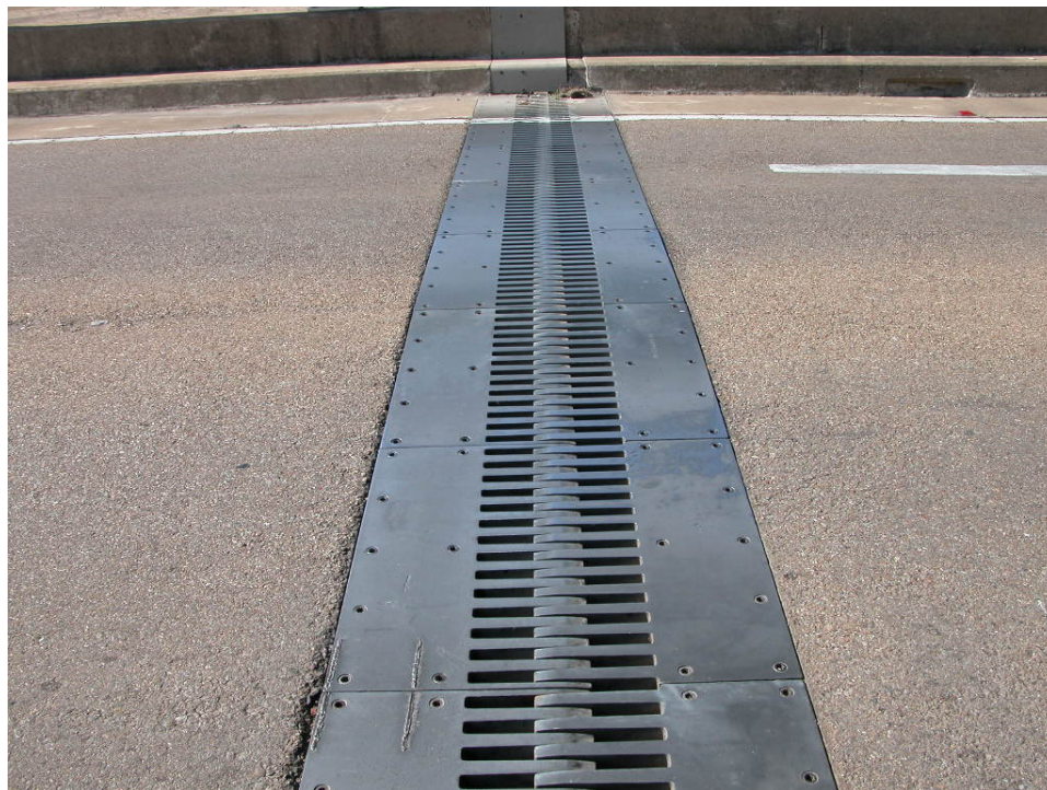
Joint in good condition.
