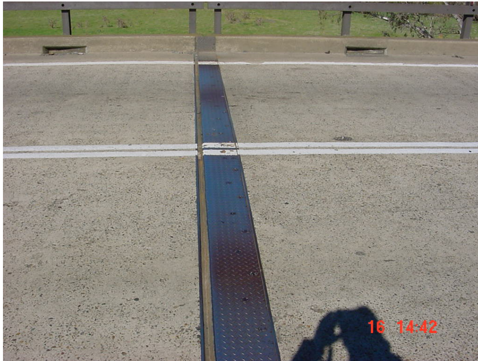
Joint in good condition.
