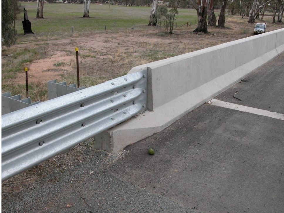
Concrete railing in good condition.
