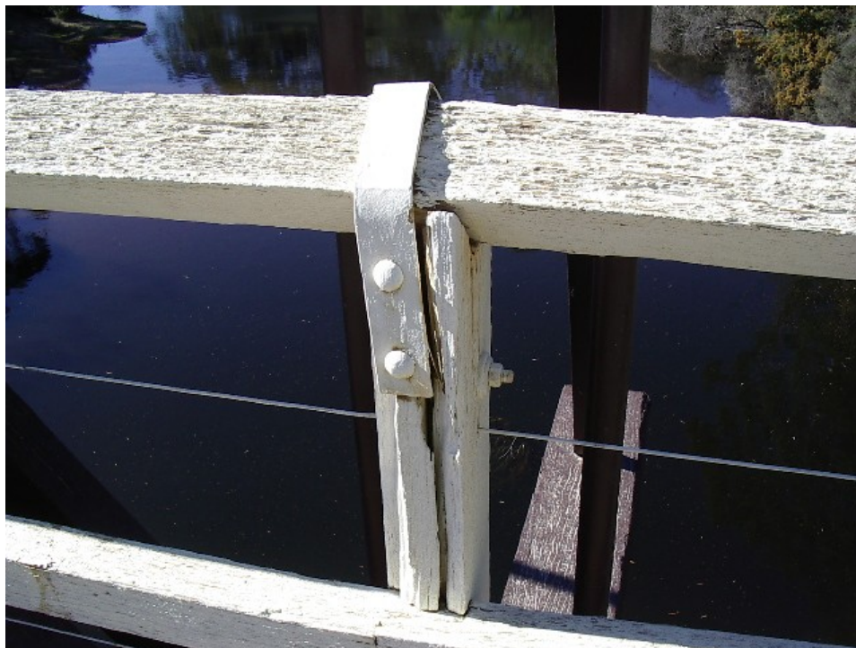
Timber railing with paint work in good condition.
