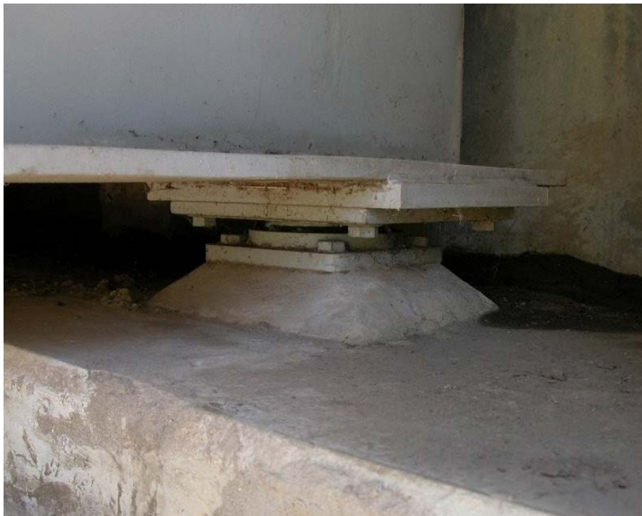
Enclosed bearing in good condition.
