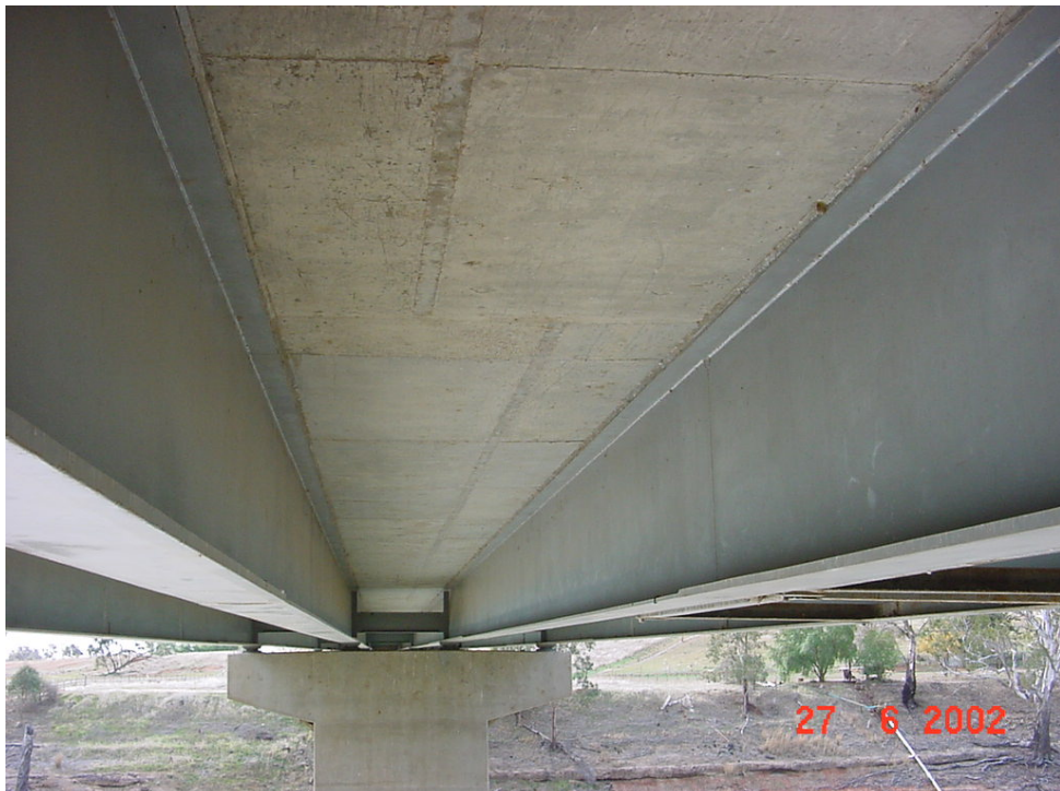
Girders in new or near new condition.
