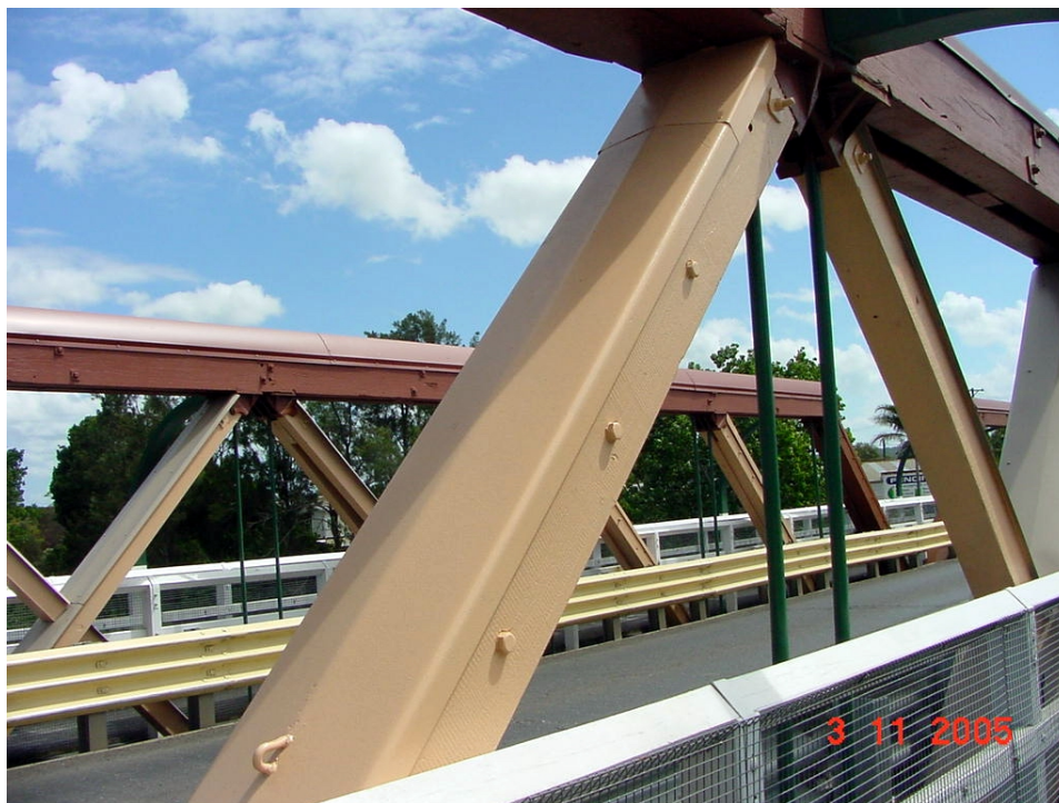
Truss paint in good condition.
