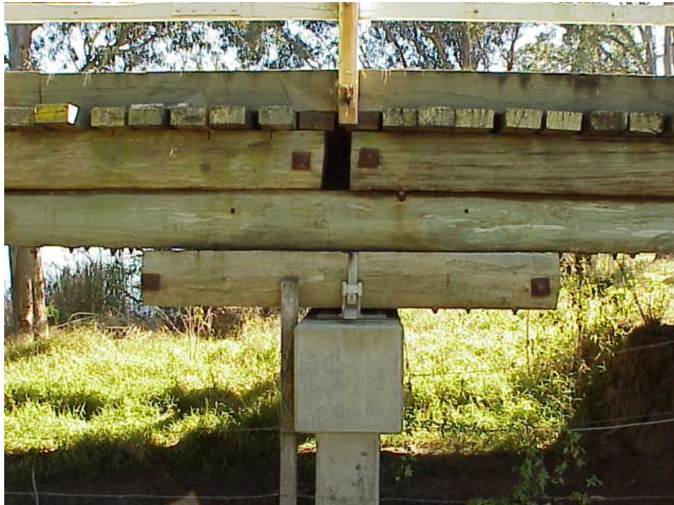
Timber corbels in good condition.
