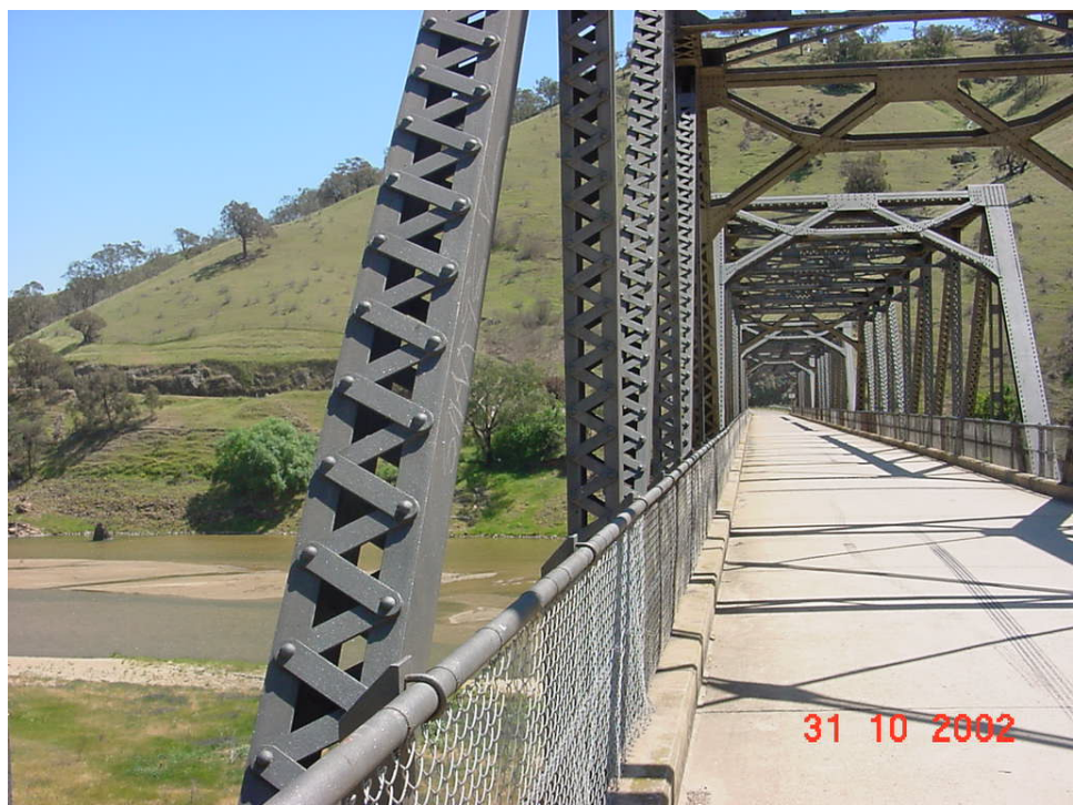
Element in new or near new condition.
