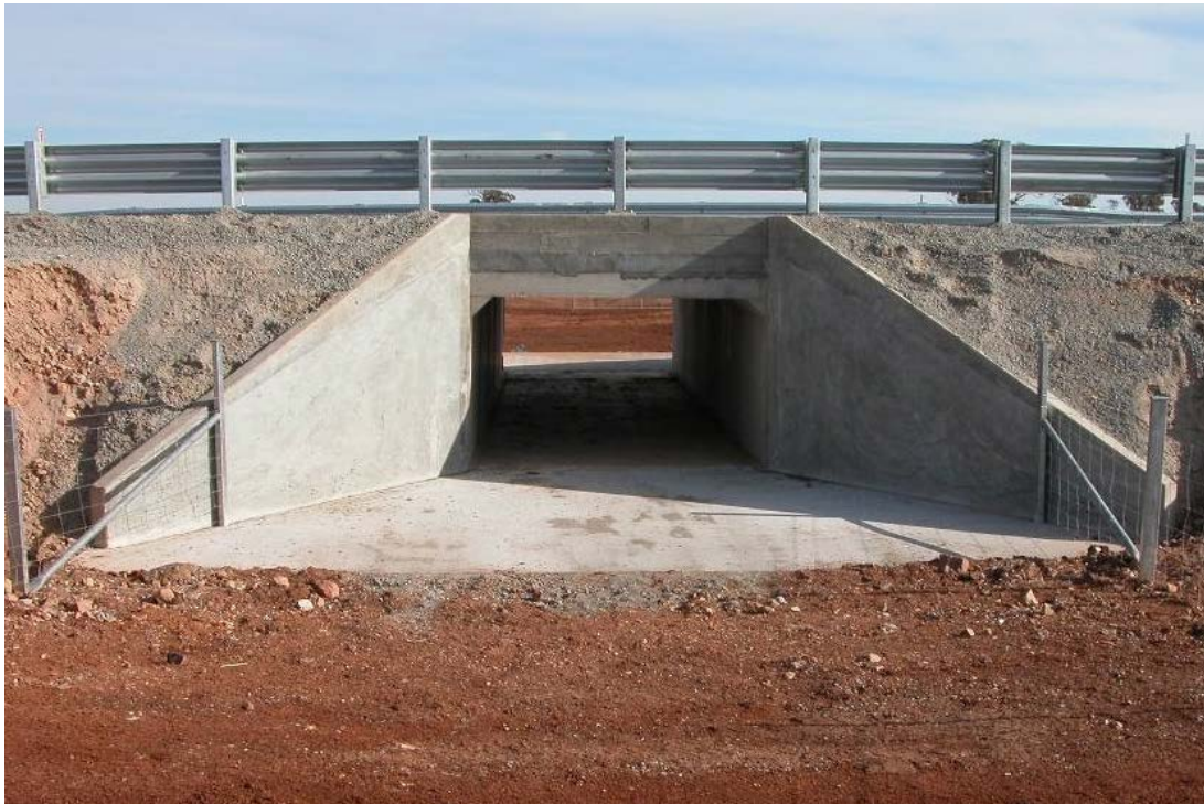
Concrete culvert in good condition.
