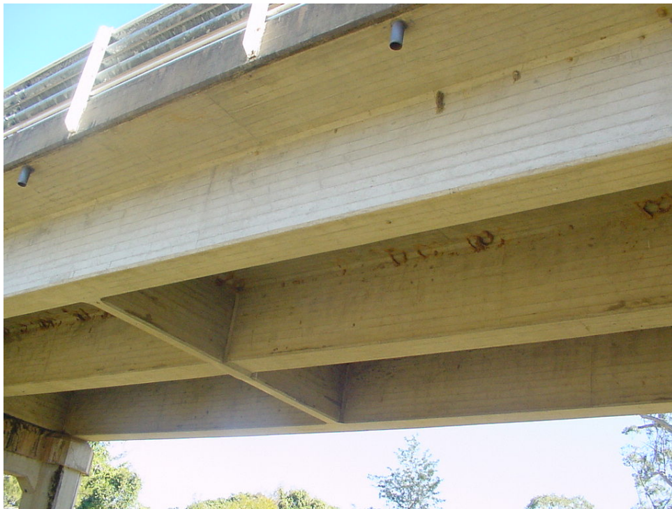
Concrete girders in good condition
