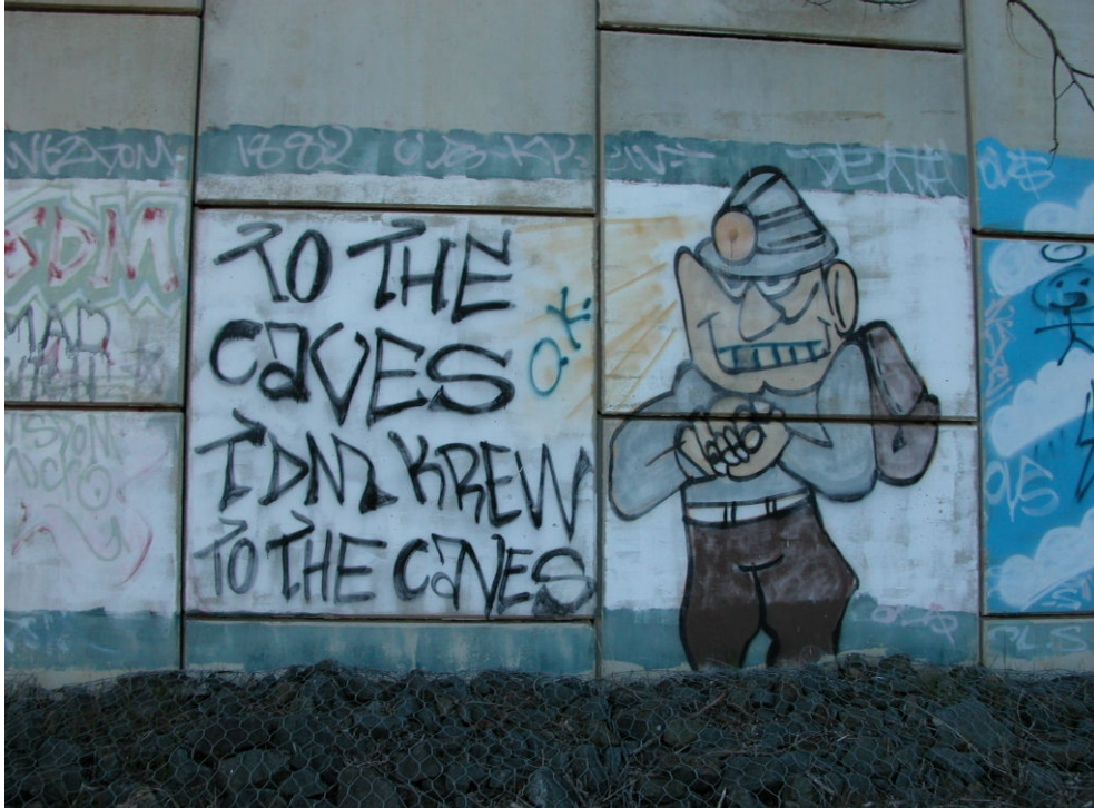
Graffiti is of some concern.
