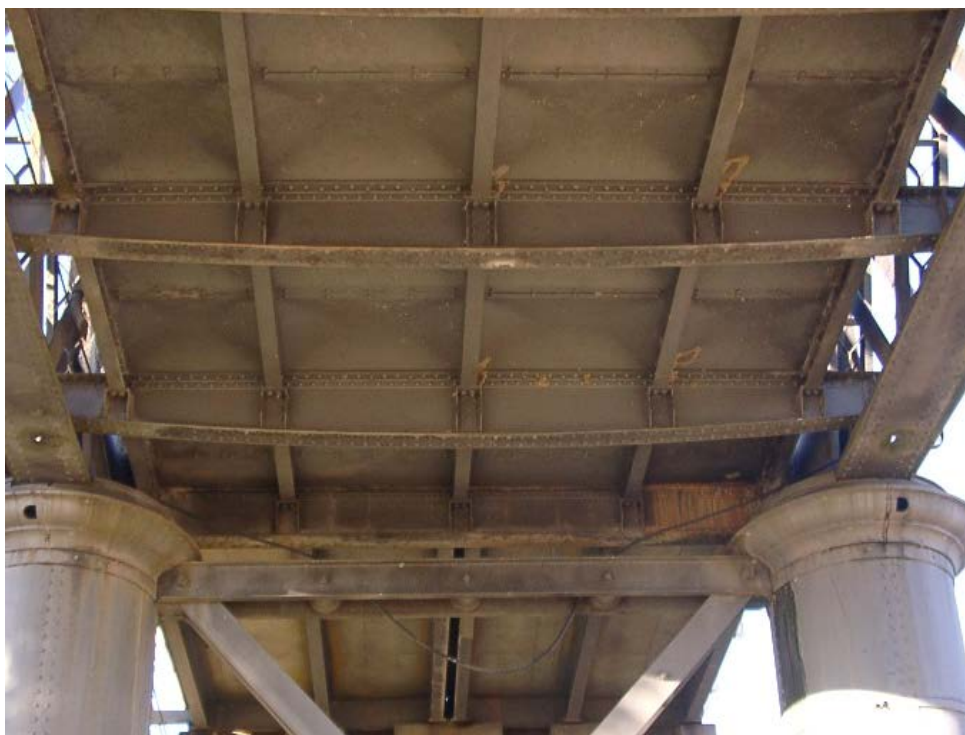
Buckle plate deck in good condition.
