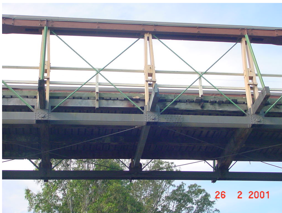
Timber truss in good condition.
