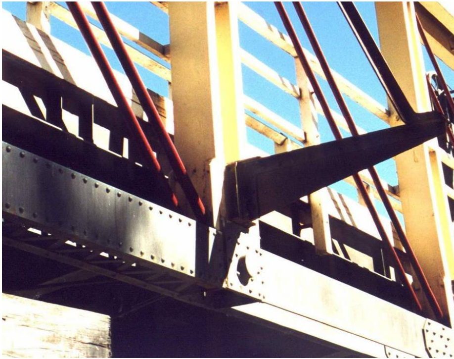
Bottom chord in good condition.
