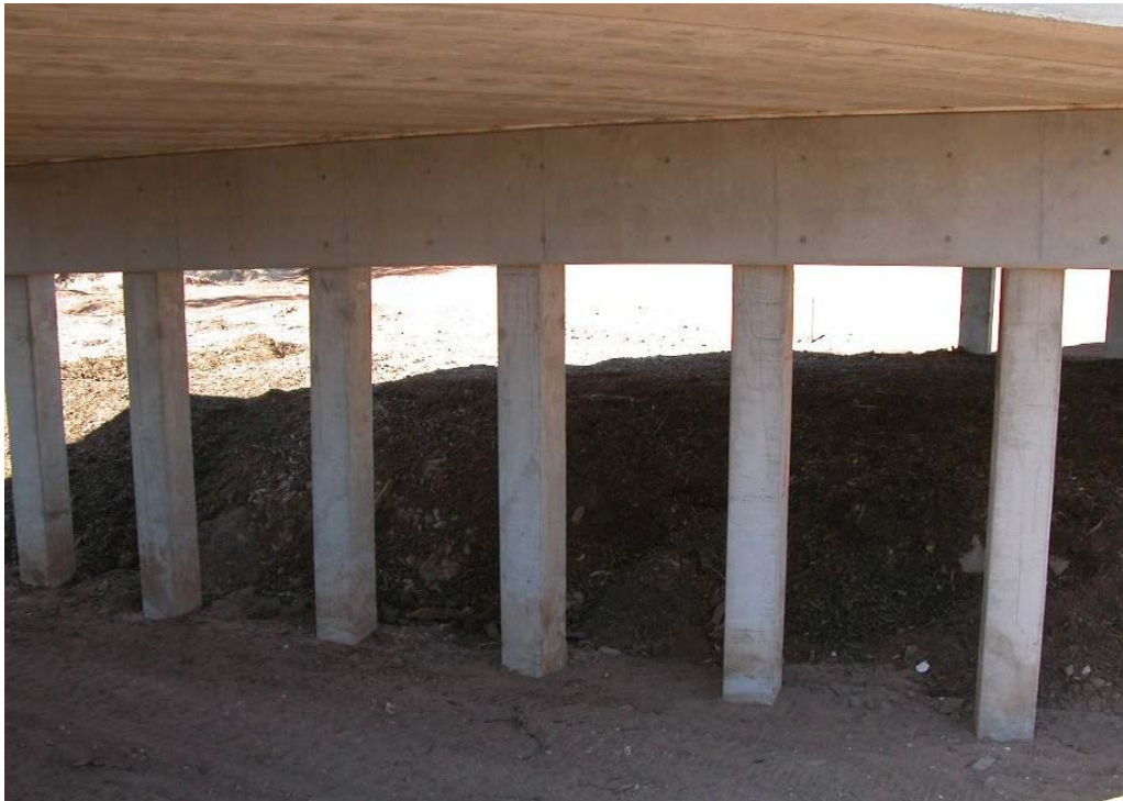
Concrete piles in good condition.
