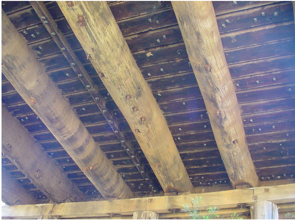
Timber girders in good condition.
