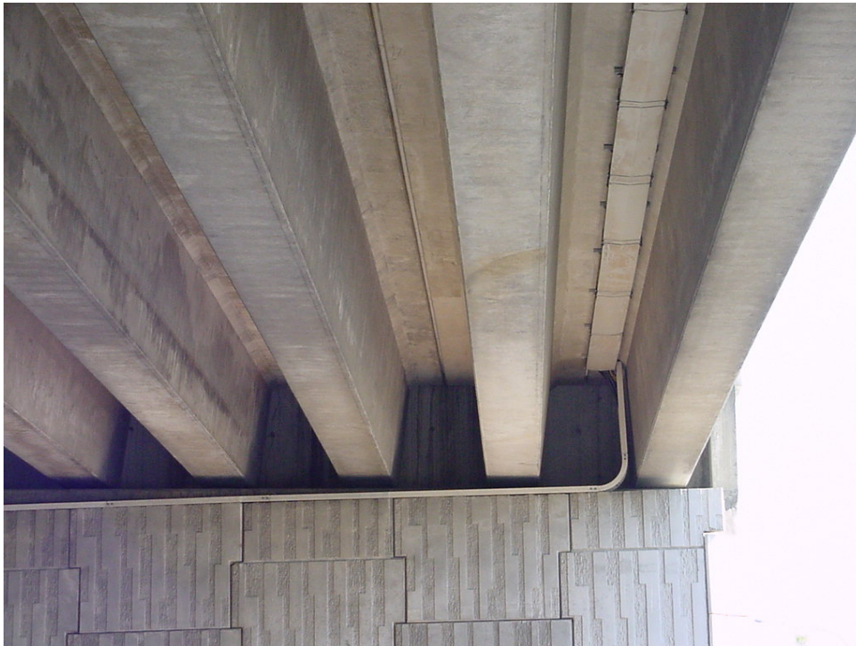
Prestressed girders in good condition
