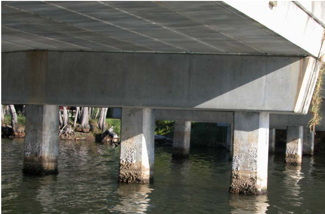
Concrete Headstock in good condition
