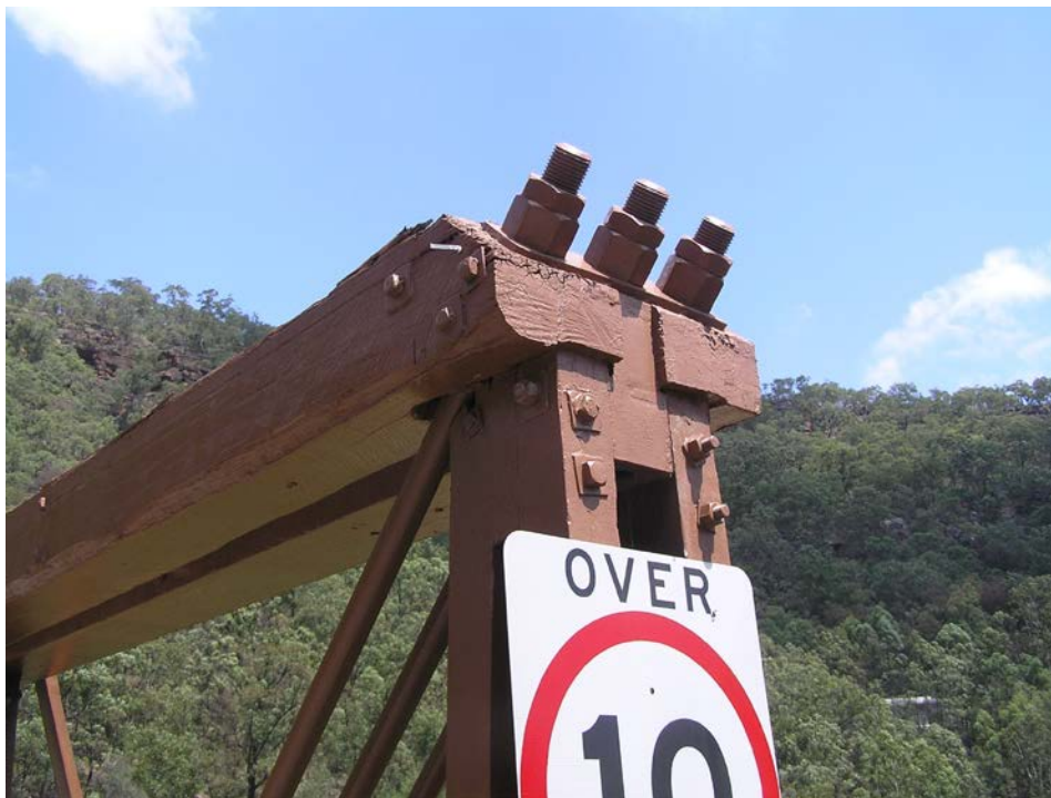
Tie rods in good condition.
