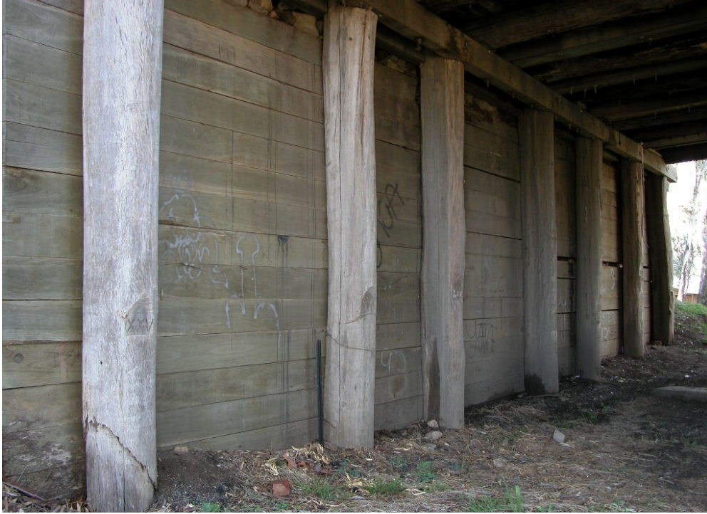
Timber piles in good condition.
