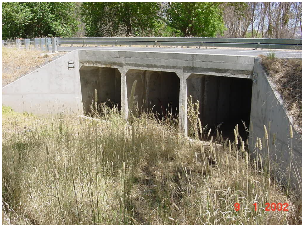
Concrete culvert in good condition.
