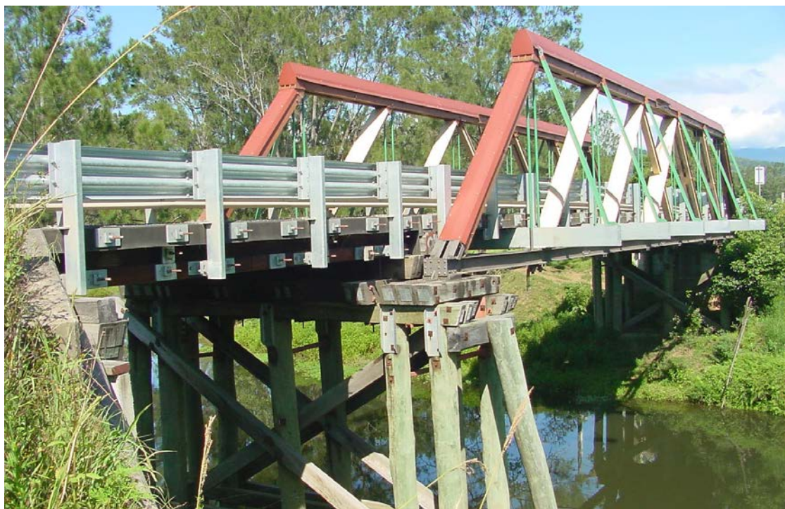
Timber truss in good condition.
