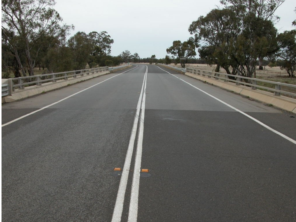
Wearing surface in good condition.
