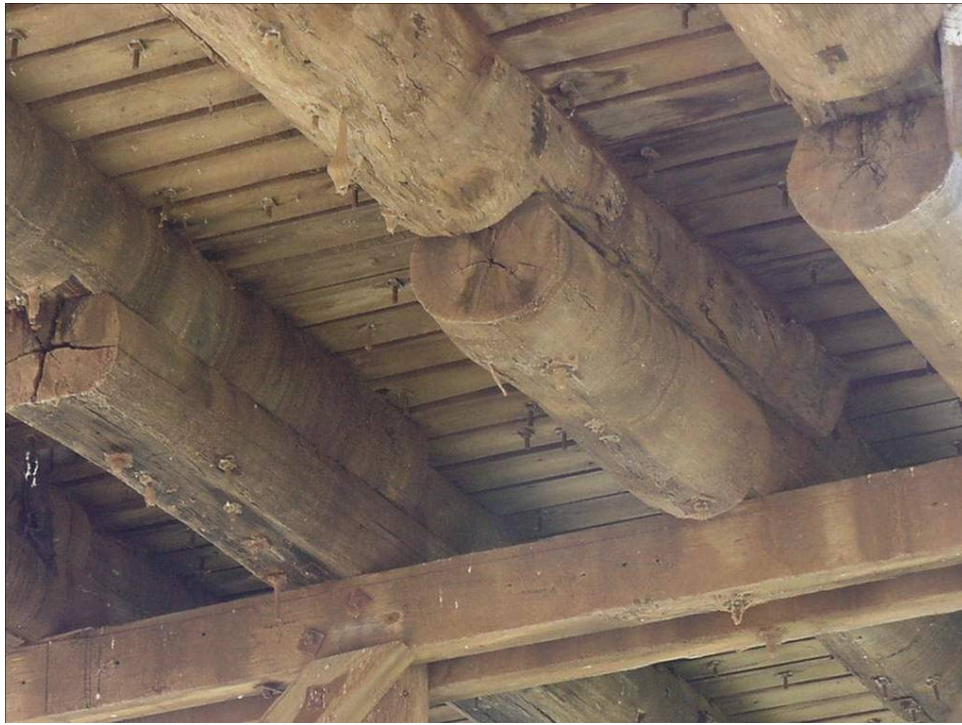
Transverse Deck planks in good condition.
