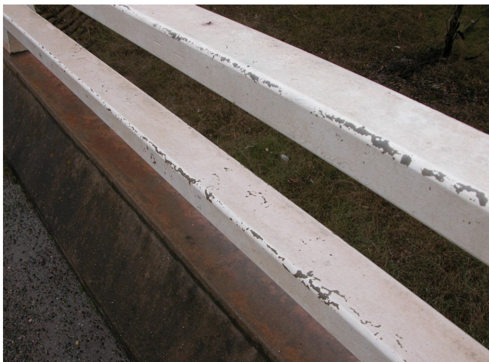
Railing in good condition.
