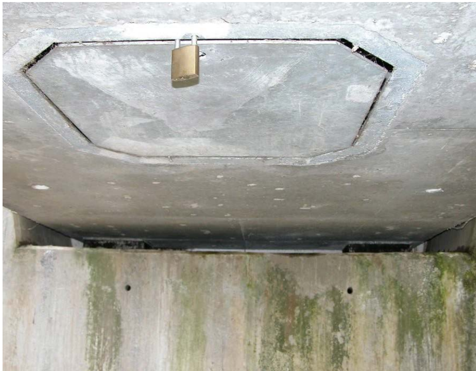
Elastomeric bearings in good condition
