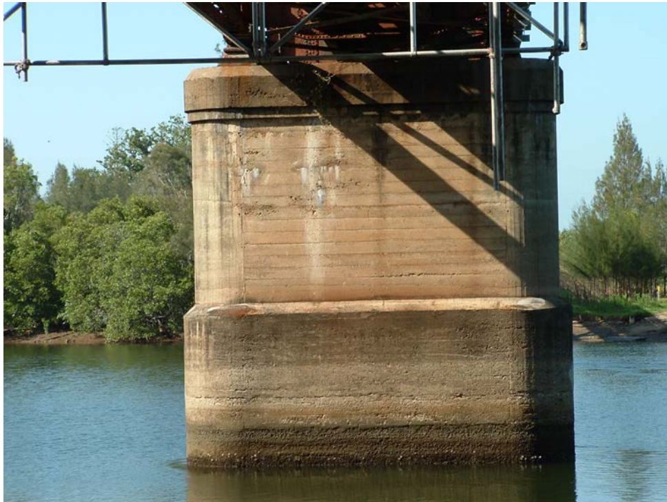
The pier in good condition with minor leaching
