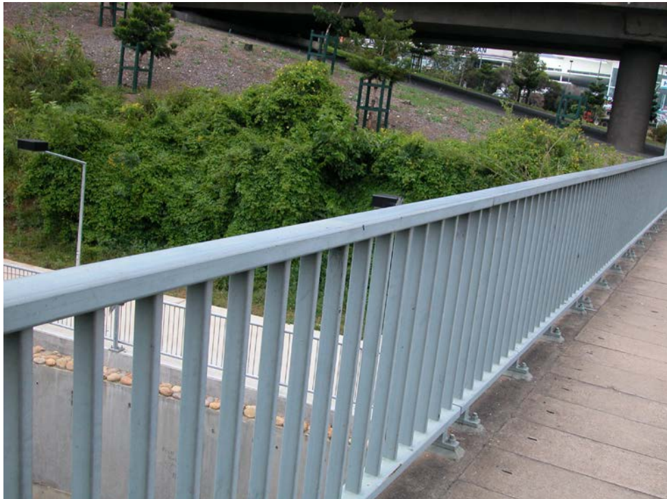
Metal railing in good condition.
