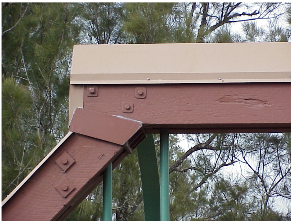
Truss paint and flashing in good condition.
