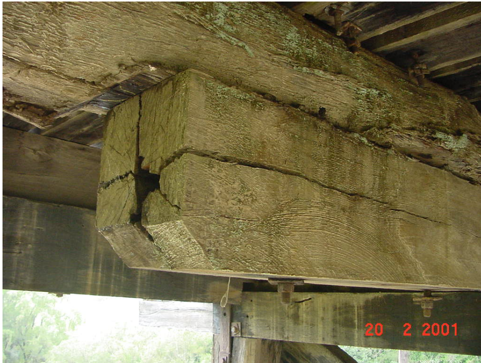
Piping with moderate horizontal split.
