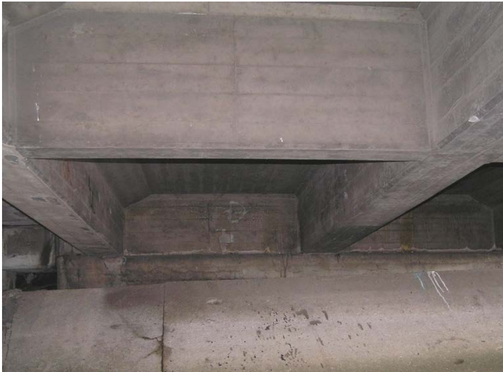
Cross girder in good condition.
