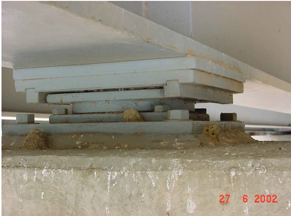
Enclosed bearing in good condition.
