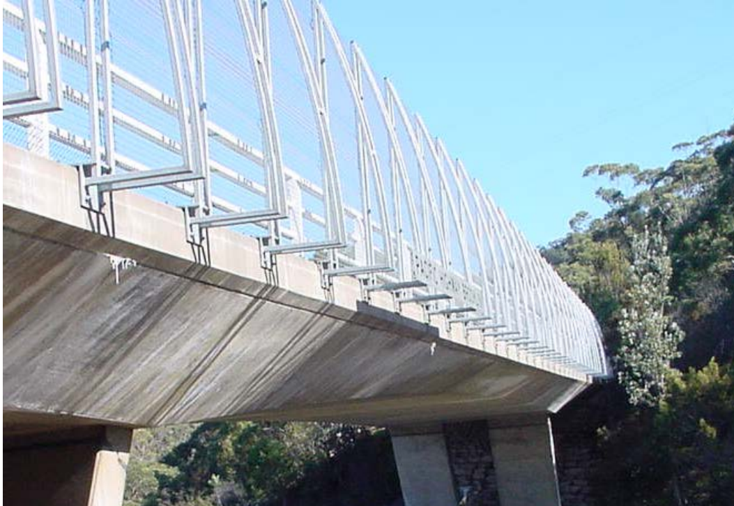
Safety screen in good condition.
