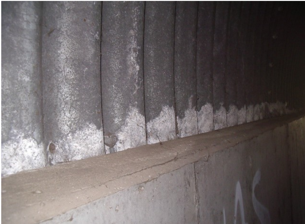
Surface discolouration near the base but culvert is still in good condition.
