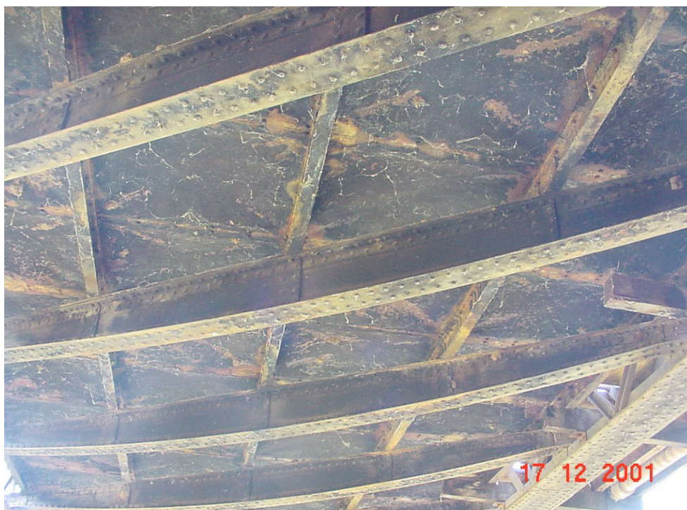
Buckle plates are still in good condition although the paint has failed.
