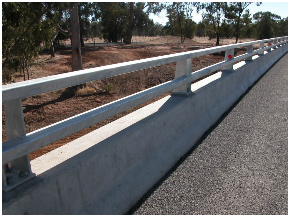
Combined railing in good condition.
